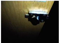
Unsuitable lock for dexterity disability
